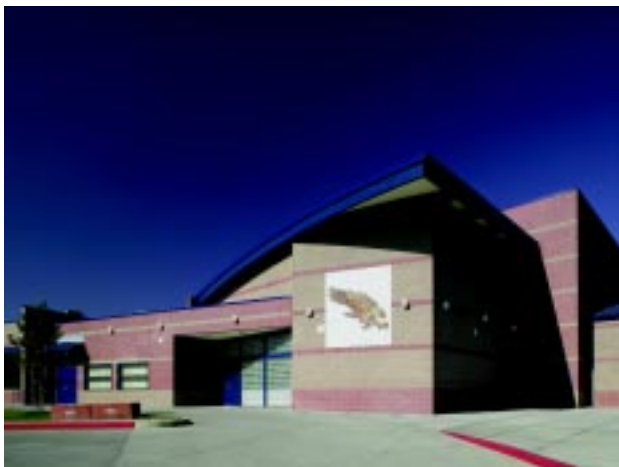
Midway High School, Dallas-Fort Worth, Texas Christopher M. Huckabee, AIA, Fort Worth, Texas
